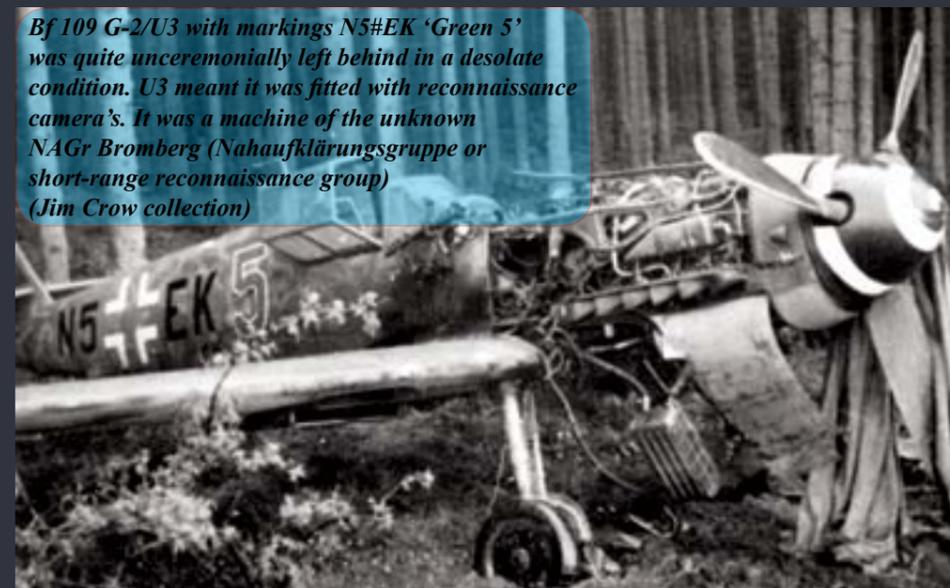
Bf 109G-2 similar to Bf 109G-1 but without pressurised cockpit. Actually, the version without pressurized cockpit was the "light version" Bf 109G-1/R2. It also had armour protection for the fuel tank removed for better performances.
